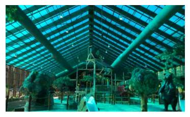
Five wall increases the R Value over traditional twin wall polycarbonate. The material is extruded with three inner layers of polycarbonate to create more air pockets, thus increasing the R Value. This makes Macrolux<sup>®</sup> Five Wall an ideal covering for all greenhouse applications where heat saving is a concern. It is also ideal for industrial and residential building such as:
